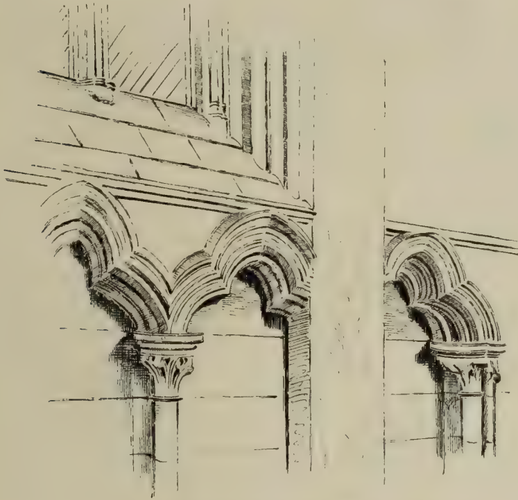
FIG. 969.—Dunkeld Cathedral. Wall Arcade at North-West Angle of Choir.
